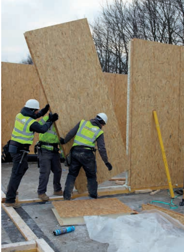
Kingspan Insulation's structural insulated panel system continues to deliver a high level of fabric performance on all projects.
