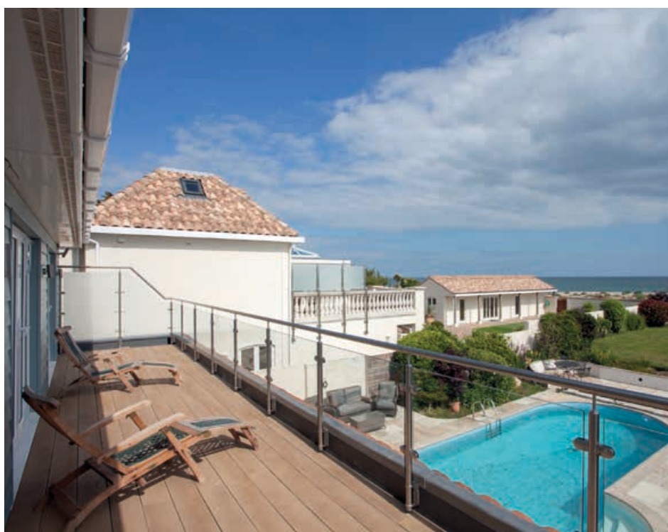
The Kingspan OPTIM-R® Balcony & Terrace System has been installed as part of the refurbishment and expansion of a four bedroom villa on the beach front in Bognor Regis.
