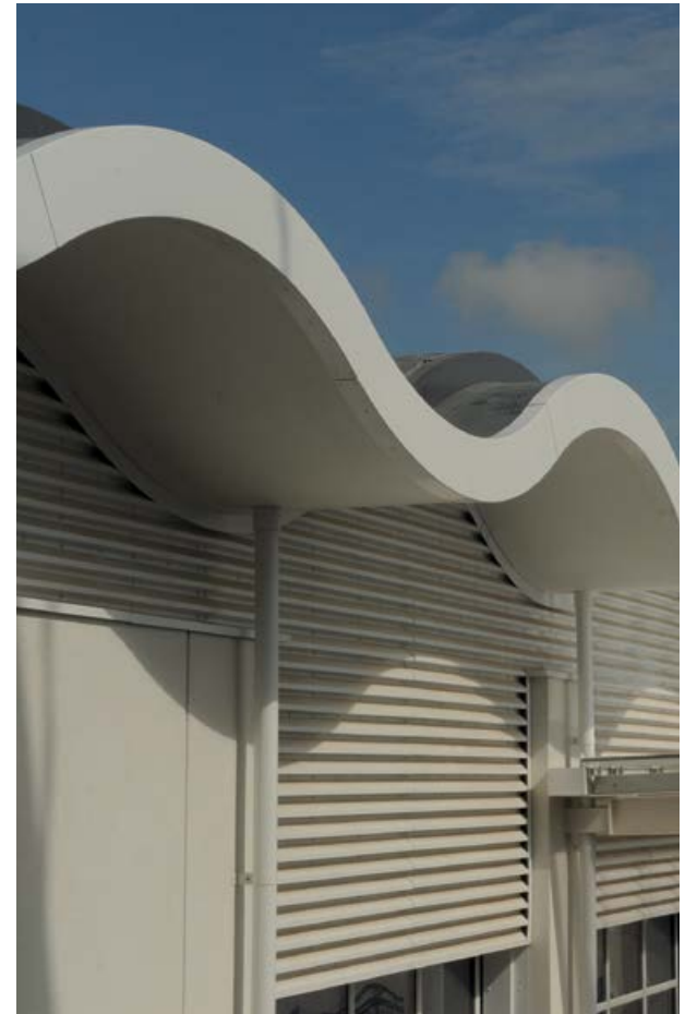
Kingspan Thermarroof TR27 LPC/FM slotted was chosen for Weymouth Fire Station's iconic wave form roof, as it provides a high standard of thermal performance, whilst also bending to the 2.5 m radius required by the roof's design.
