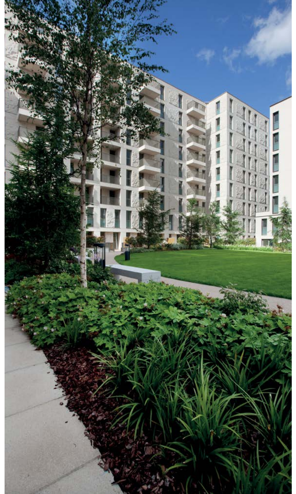
Kingspan Kooltherm K15 was installed as part of the London Olympics Athletes Village. Picture source ODA.
