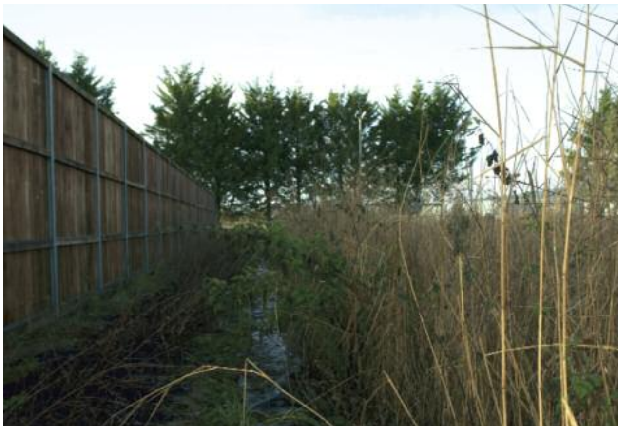
The reed bed at Pembridge continues to operate effectively.
