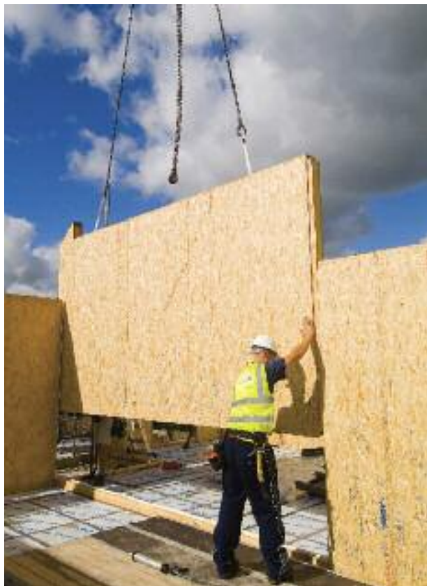
The Kingspan TEK Building System uses structural insulated panels that hitherto have been manufactured near Berlin and shipped to the UK. This manufacturing process is to be moved to Selby during 2012.
